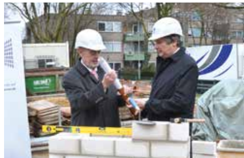
Laying the foundation stone for the new part of the building on 27 February 2015
